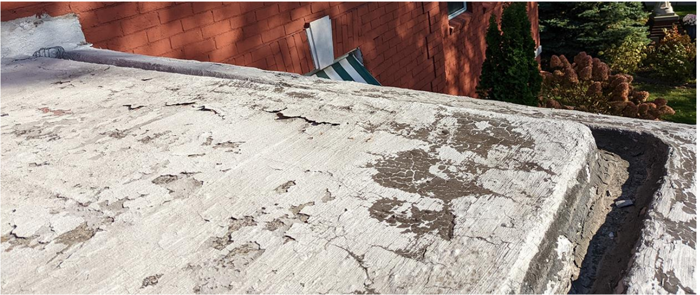
Existing condition of porch roof. Photo provided by applicant.
