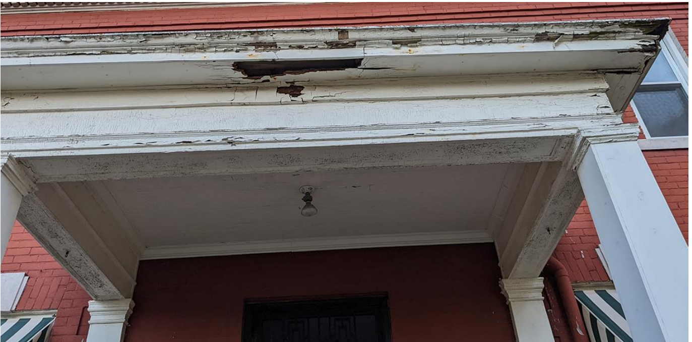
Existing condition of porch. Photo provided by applicant.
