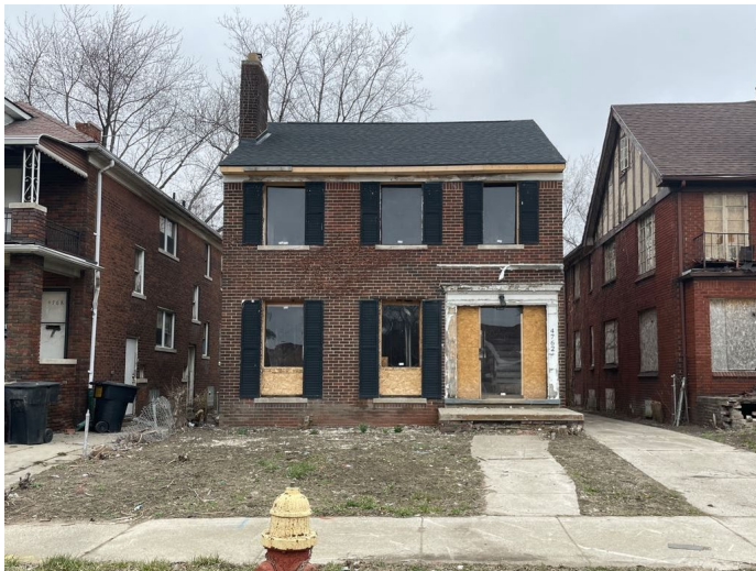
Site Photo 1, by Staff March 22, 2023: (South) front elevation.
