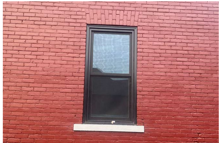
Site Photo 4, by Applicant 2023: (East) side elevation showing new installed window flush with wall opening.
