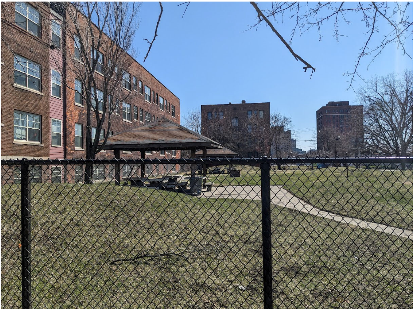
View of existing conditions at 469 Brainard, looking towards the south. Staff photo, March 30, 2023.
