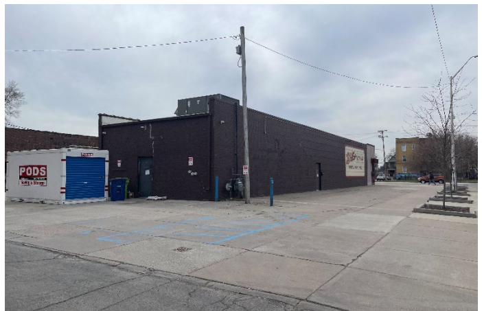
Site Photo 2, by Staff March 24, 2022: (Northeast) side elevation and adjacent lot, showing location of proposed patio roof structure.
