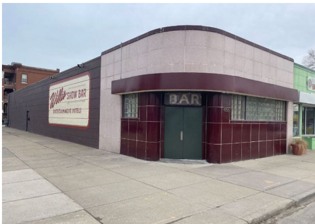
Site Photo 1, by Staff March 24, 2022: (Northwest) front elevation
