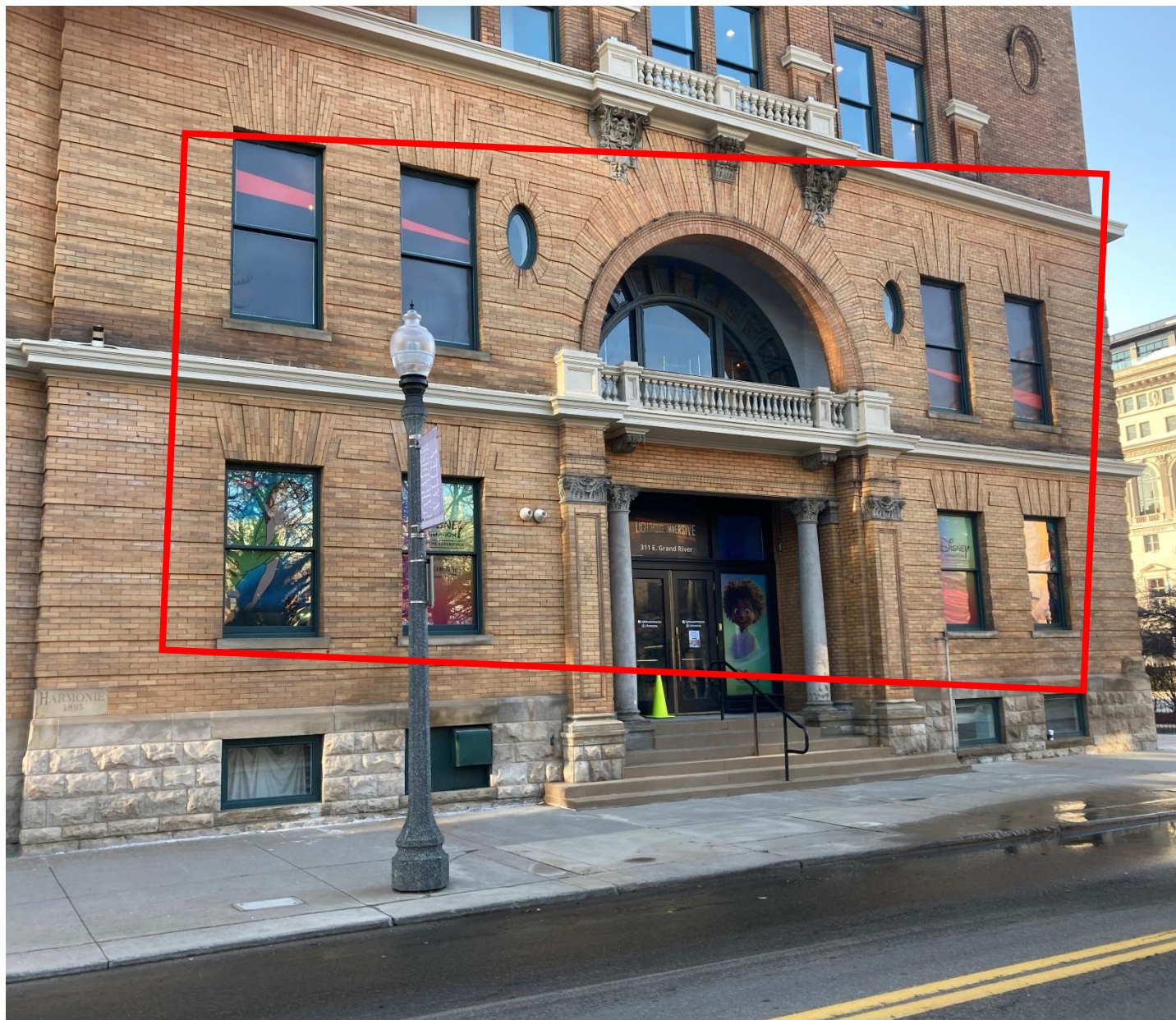
The subject signage which was approved by HDC staff for temporary installation within the eight double-hung windows and the front doorway within the sidelites and transom. This signage is the subject of the current application. Staff photo taken on 2/28/2023
