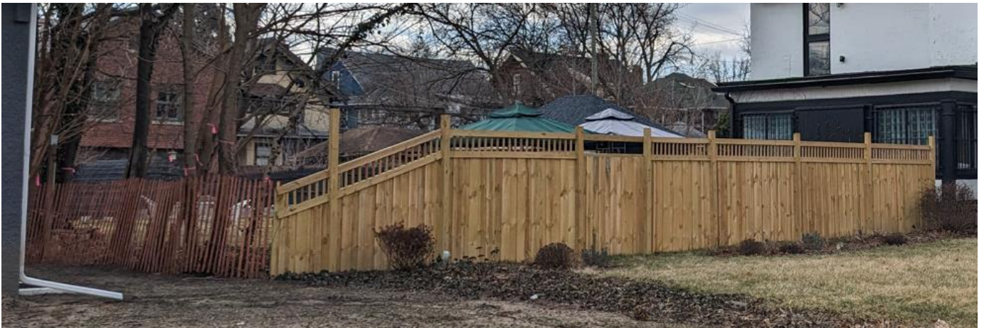
Eastern termination of the fence. February 2023 site visit photo by staff.
