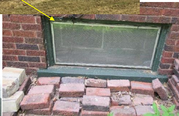
Fig 12: Typical original basement window
