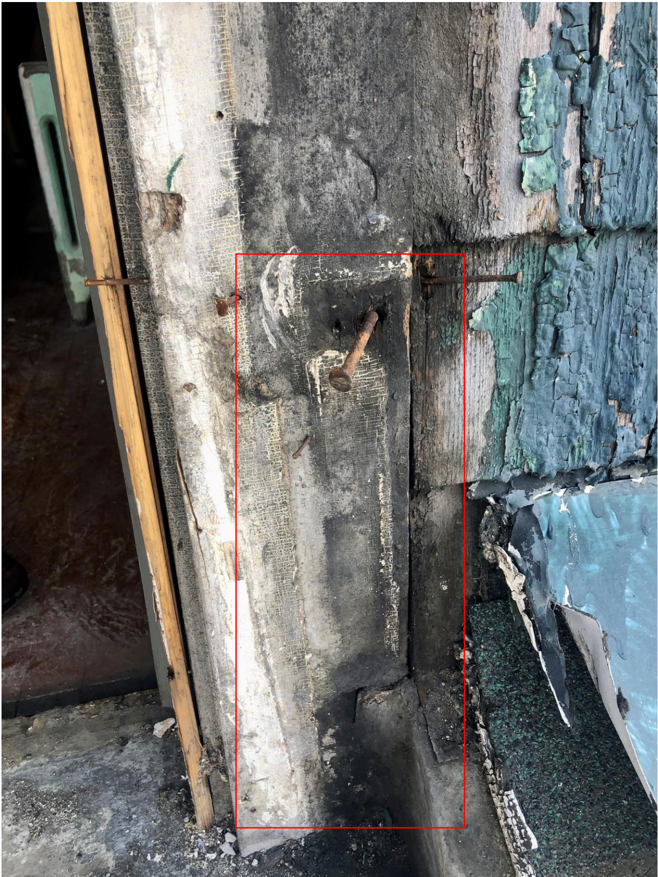
Staff photo, March 6, 2023. Some visual evidence of the upper porch railing is evident.
