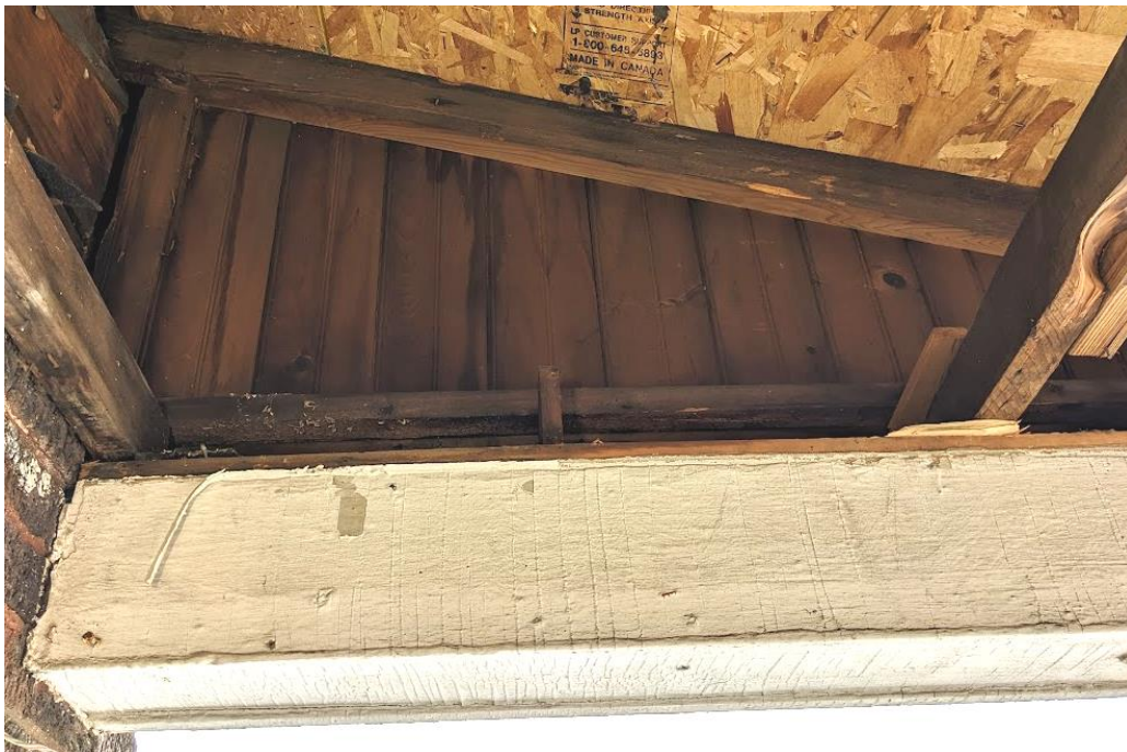
Staff photo, March 6, 2023 - interior of gable wall supporting the shed roof.
