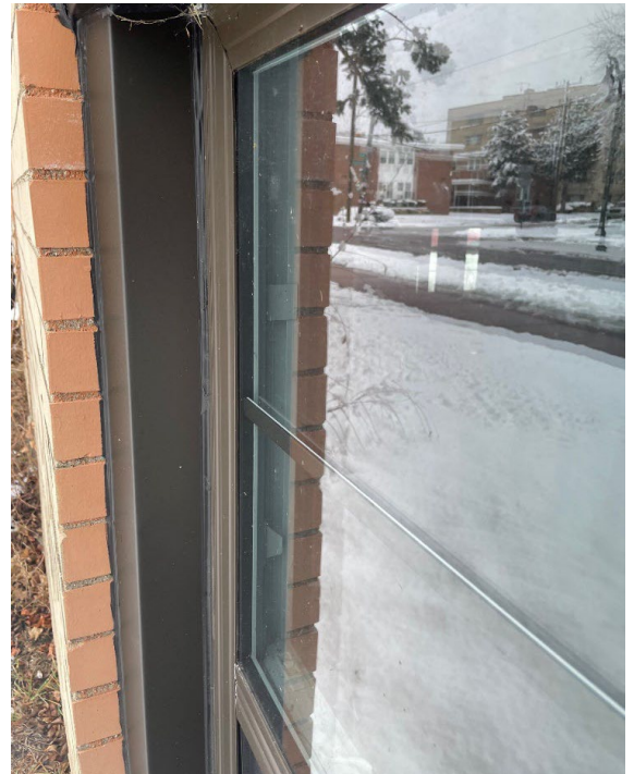
Detail photo 1, by applicant: Third street (west) front elevation, showing where original brick mould was replaced with aluminum brick mould and horizontal muntin between the glass
