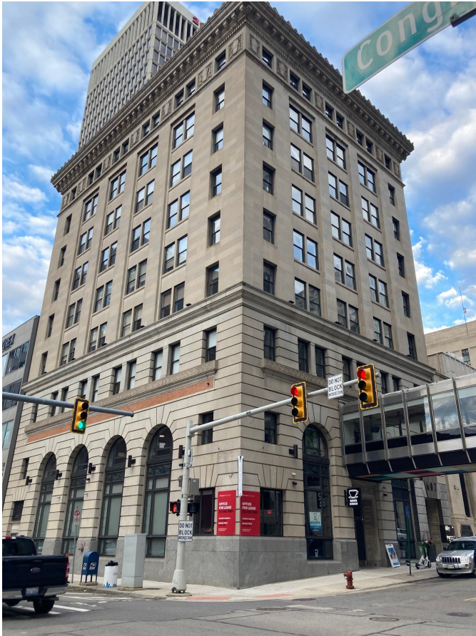
Figure 1. View of 607 Shelby St. looking northwest.
