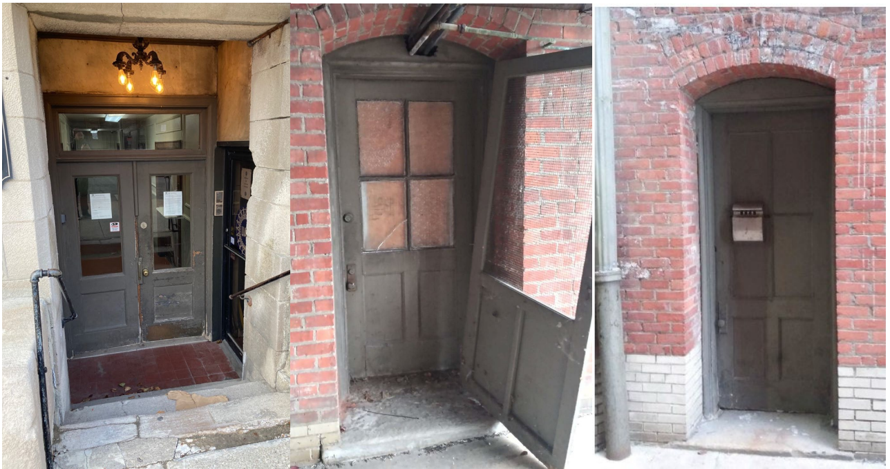
Figure 5. L-R: Storefront door, typical fire escape door, courtyard door.
