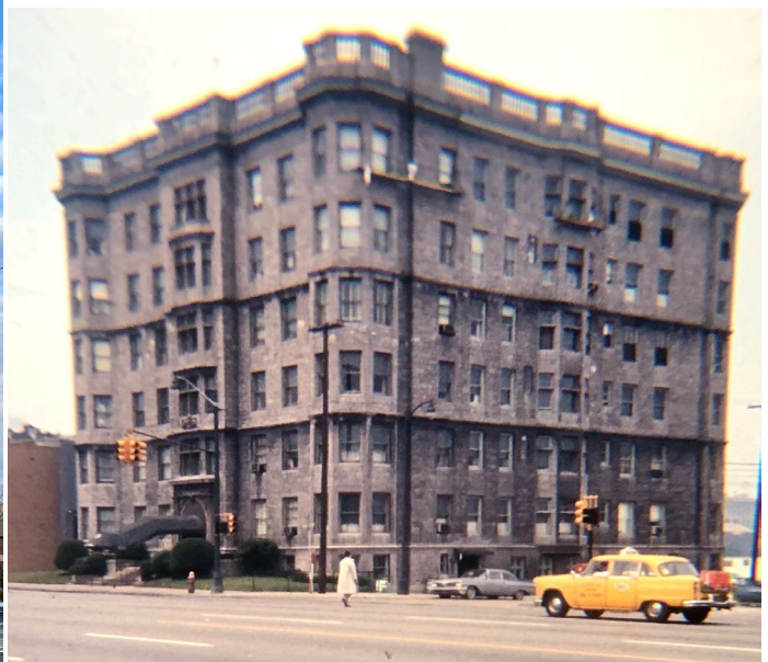
Figure 2. Ca. 1980 photo of the Palms Apartments. HDAB.
