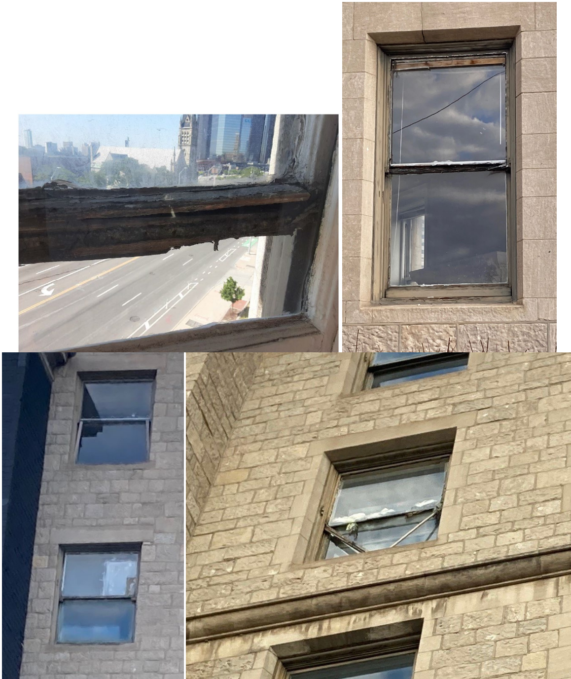
Figure 3. Examples of existing conditions of the wood double-hung windows
