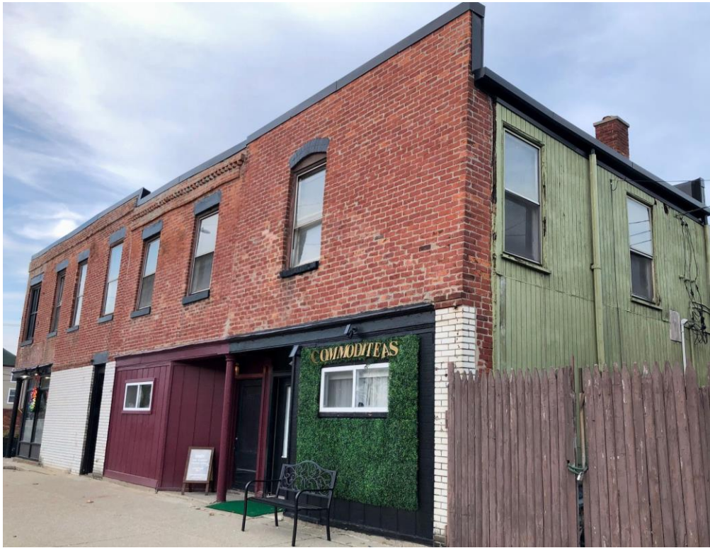
Trumbull elevation looking northeast. Staff photo, November 29, 2022
