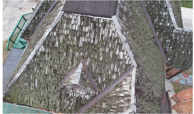
Roof Detail 2, by MGS inspection: Exterior roof conditions.
