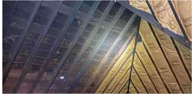
Roof Detail 1, by Schaufele inspection: Interior roof conditions.
