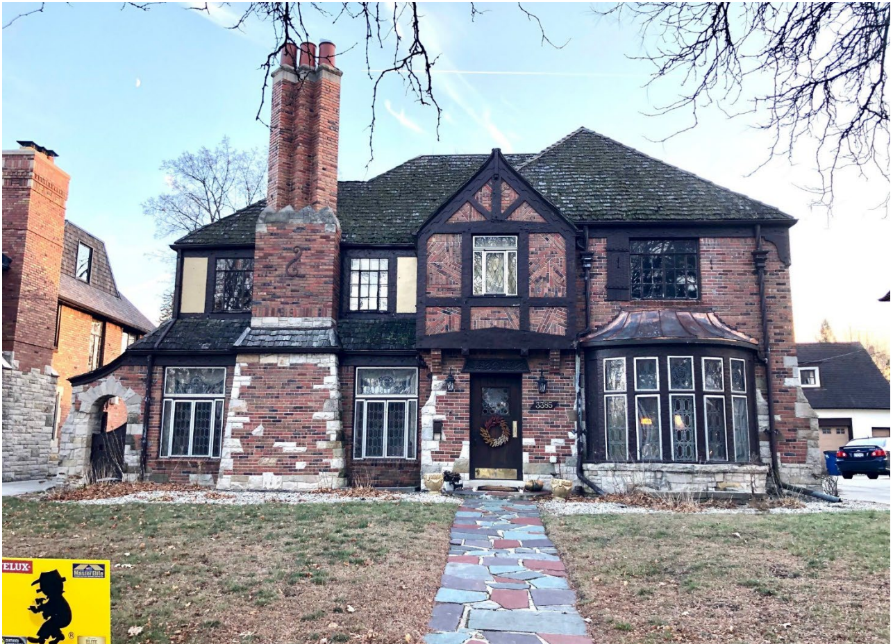
Site Photo 1: Staff photo, November 29, 2022
