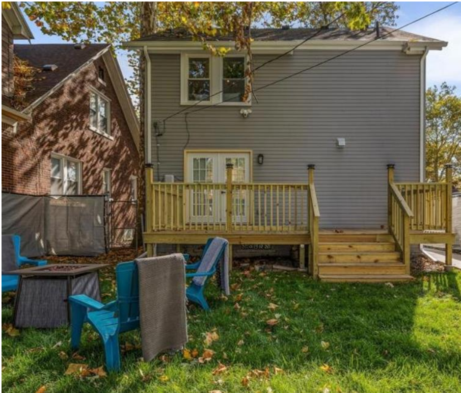
4370 Glendale, current appearance of rear elevation (source - realty.com 4370 GLENDALE, Detroit, MI 48238, MLS# 60155412 - mimc (realty.com) )
