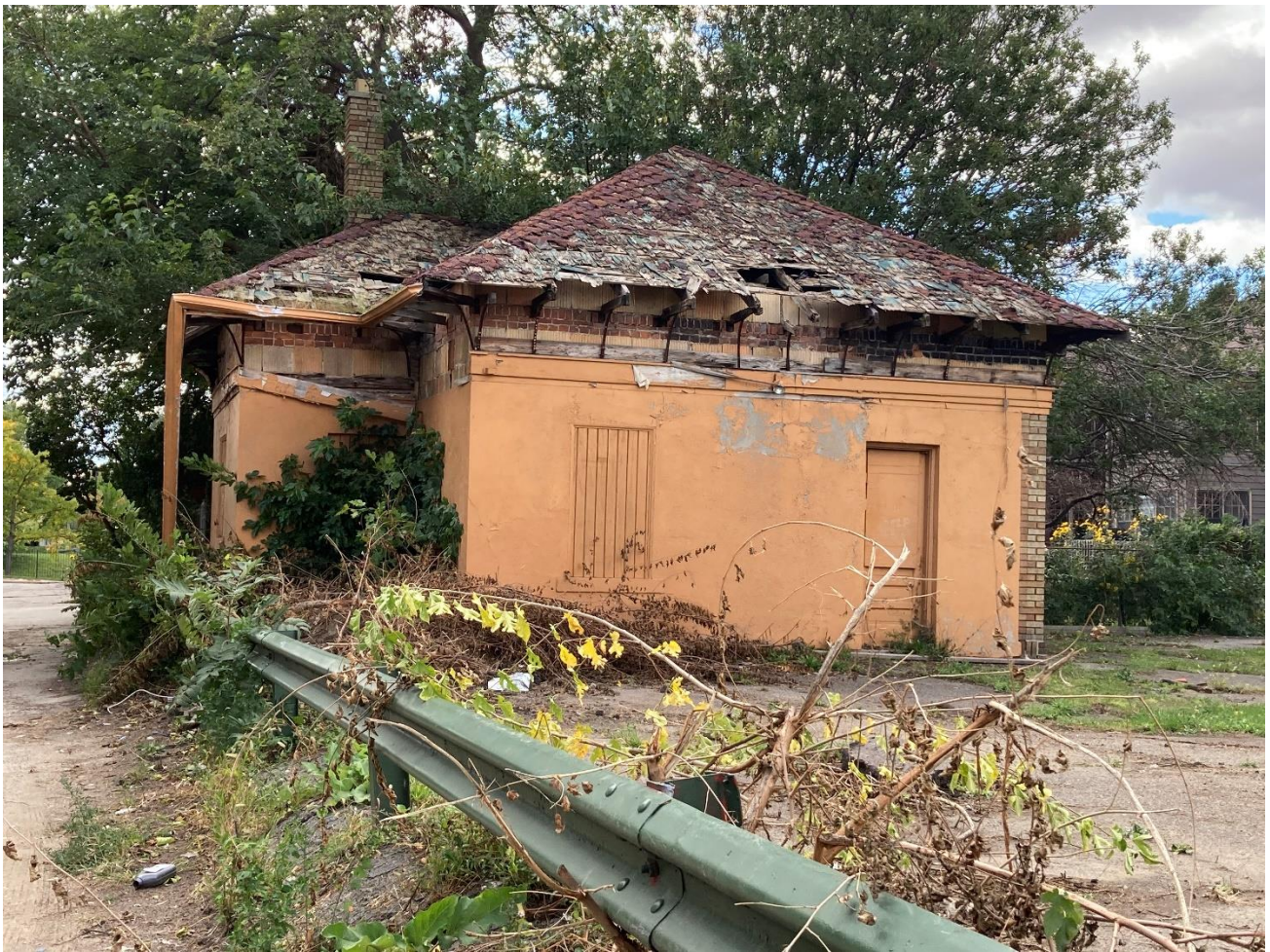
873 Virginia Park garage, current appearance (staff photo taken 12/1/2022)
