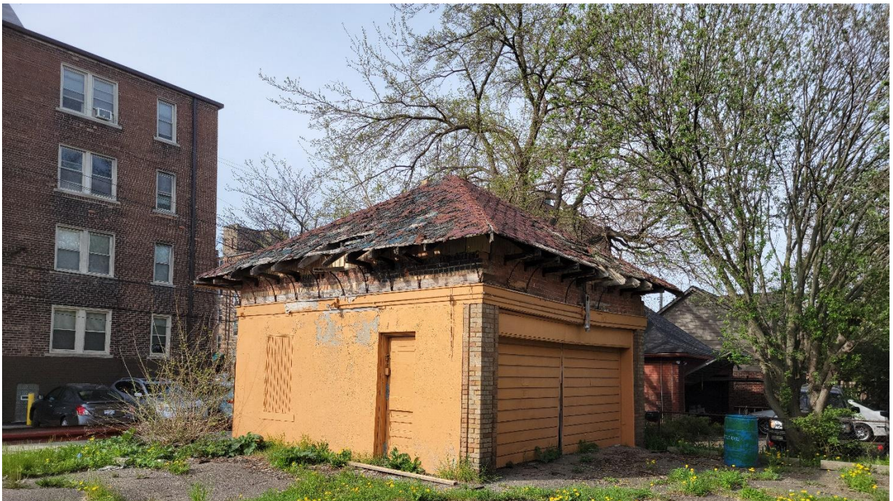
873 Virginia Park garage, current appearance (applicant photo submitted 9/2022)
