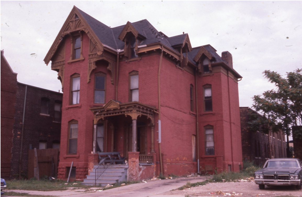
HDAB Designation Photo of 291 Winder, 1980. The original nineteenth century three-story mansion featured red brick and a spectacularly intricate and ornamented roof line and porch. Note the early twentieth century apartment block addition extending to the rear, a typical addition in Brush Park to accommodate more residents in the twentieth century.
