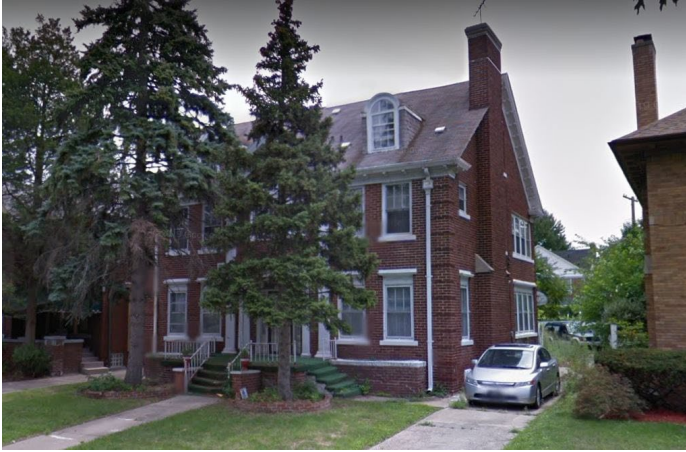
Site Photo 3, Google Streetview Aug. 2011: (Northwest) front/side elevation showing front porch alterations made with added wingwalls to front steps. Planter boxes on either side are still in place.
