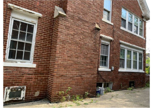
Site Photo 7, by Applicant: (West) side elevation showing original wood windows.
