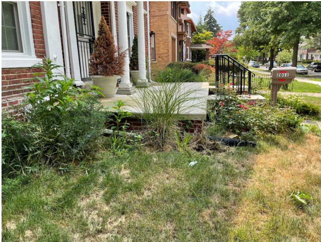
PORCH - SIDE (EAST) ELEVATION
