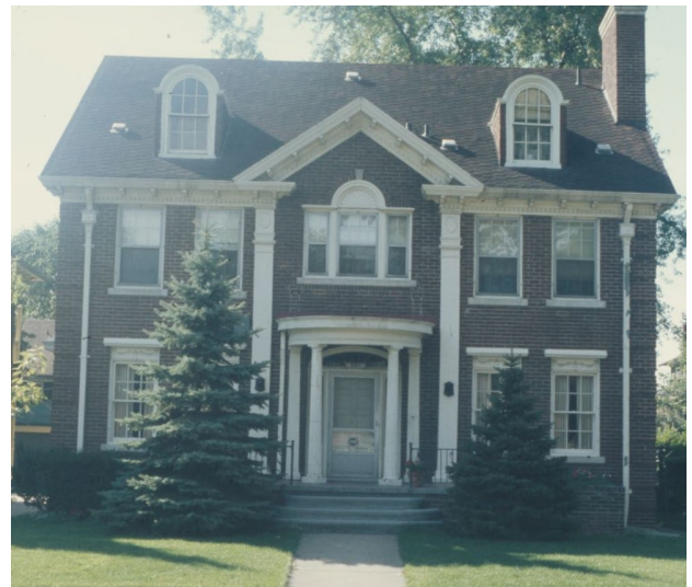
Site Photo 2, designation slide 1980: (North) front elevation.
