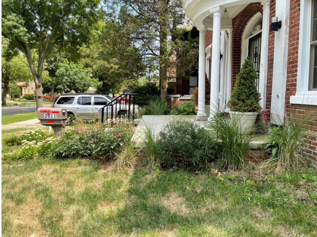
PORCH - SIDE (EAST) ELEVATION
