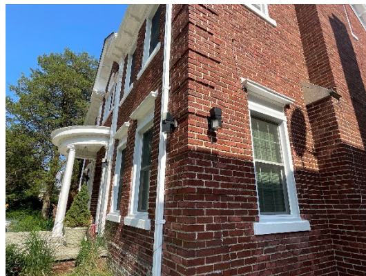
Site Photo 8, by Staff: (Northwest) front and side elevations showing locations of security lights at on the brick quoins and front pilasters of the house.
