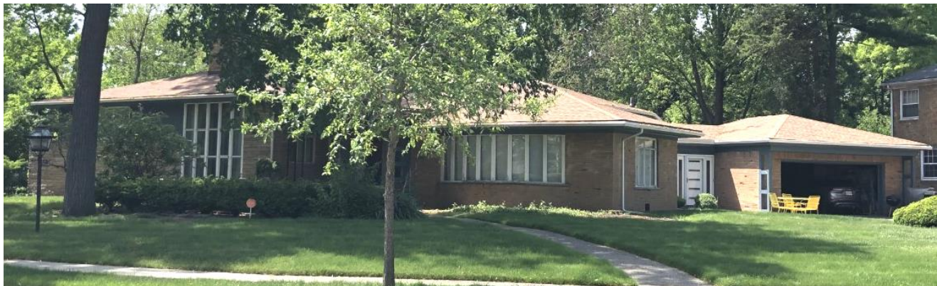
Looking northwest from Parkside at front and east elevation. HDC staff photo, May 2021.
