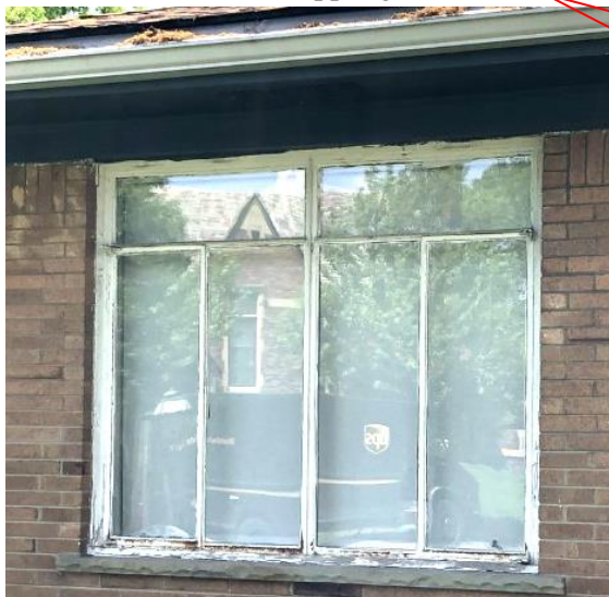
Original steel window, Staff photo, May 2021
