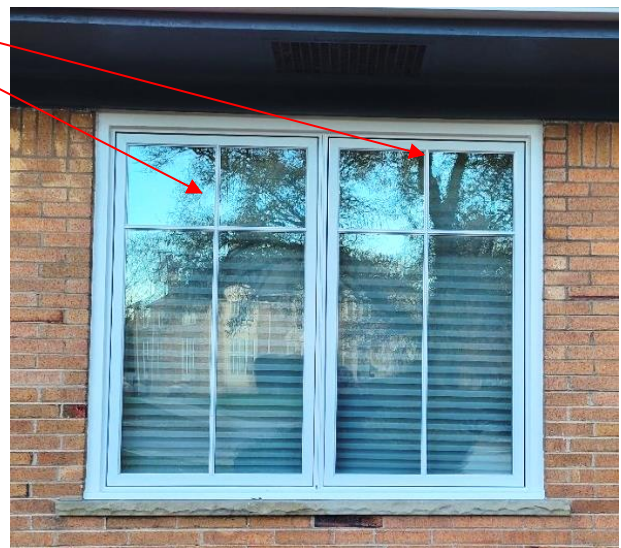
Replacement window, Applicant photo
