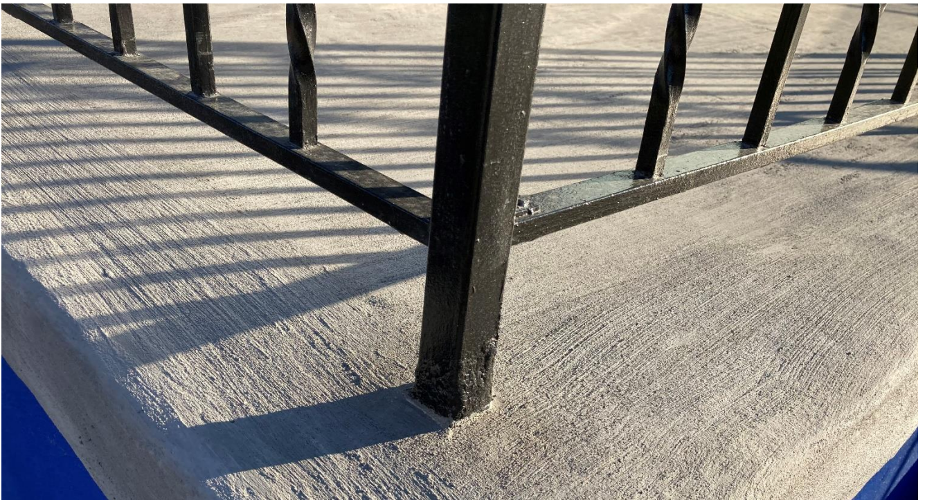
2648 W. Grand Blvd, current conditions. Staff photos taken 9/9/2022
