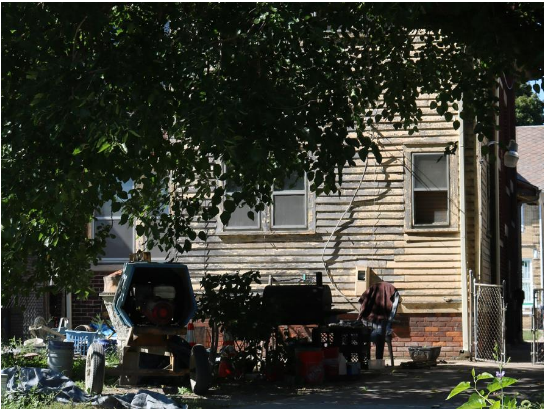
Rear (south elevation) of building. September 2022 photo by staff.
