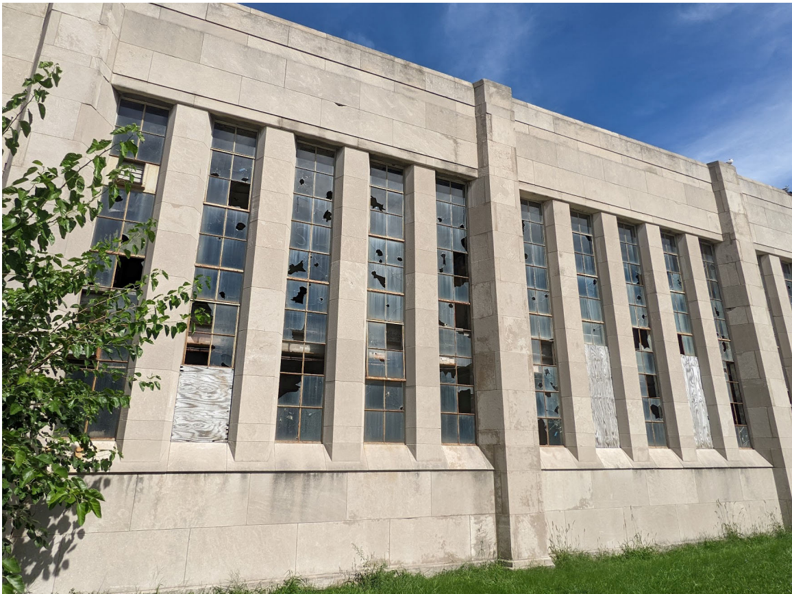
View of East Elevation (north block). Staff photo, 9/2/2022.
