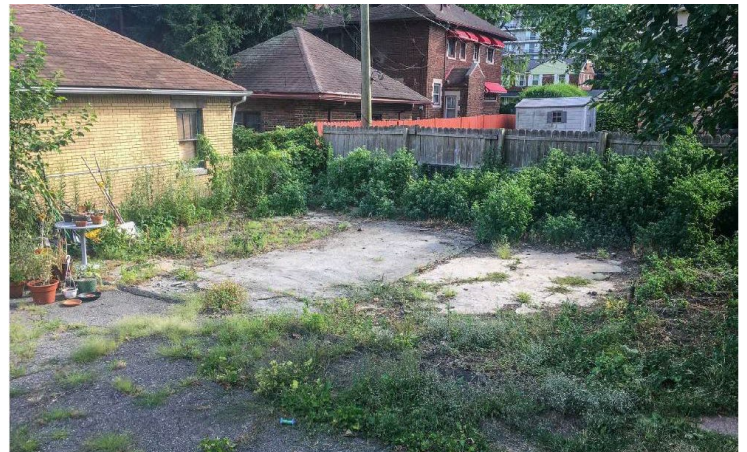
Site Photo 2 by Applicant: (South) rear yard, showing current condition of garage site, demolished by former owner.
