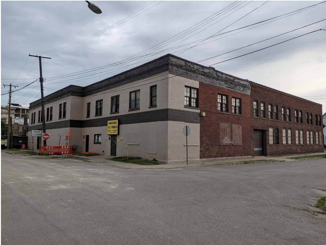
View of 1567 Church, looking southeast from intersection of Church and 10th. Staff photo, July 1, 2022.
