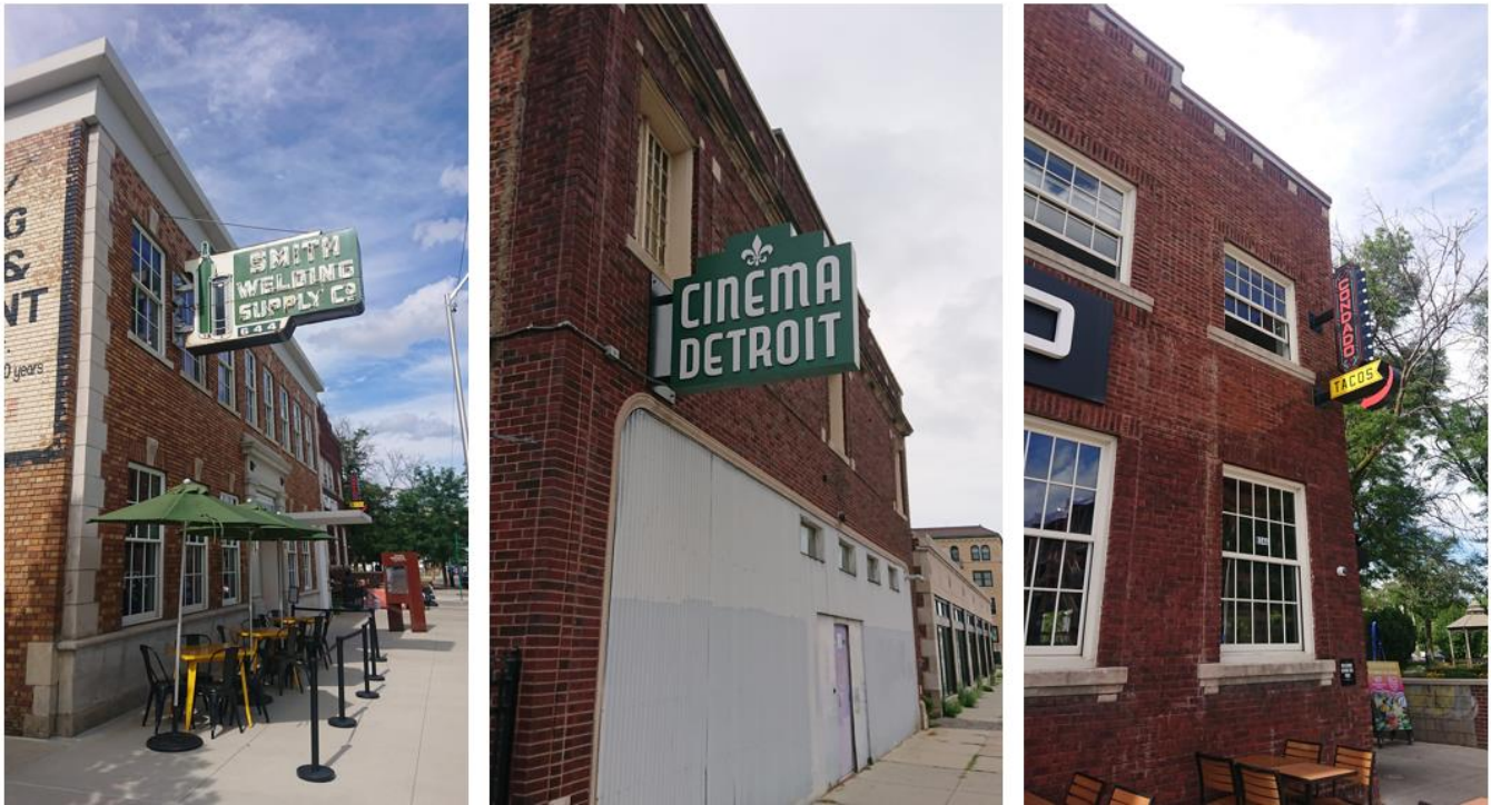
Comparable projecting signs in Willis-Selden. Left: Historic. Center and Right: Certificate of Appropriateness. July 2022 photos by staff.
