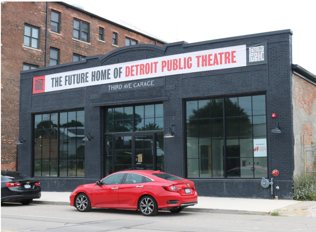
View from Third St. looking east towards west façade of building. July 2022 Photo by staff.
