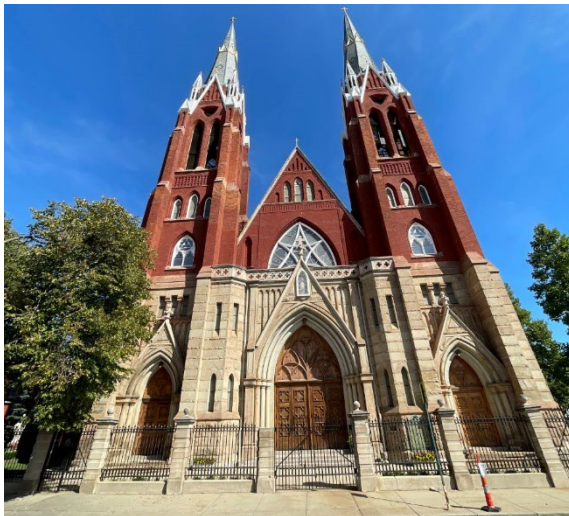
Front of Church (West)
