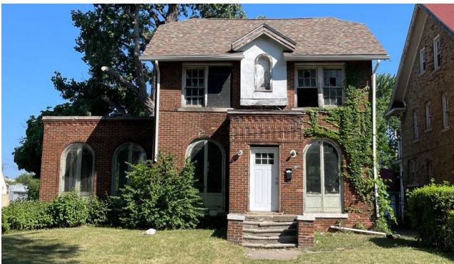
Site Photo 1, by Staff July 21, 2022: (North) Front elevation.
