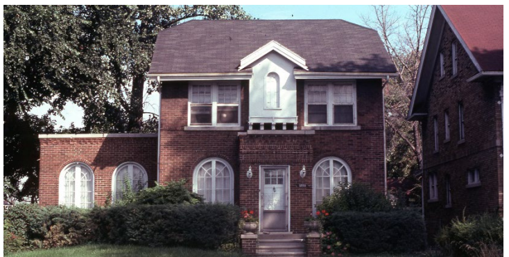
Site Photo 2, designation slide 1974: (North) front elevation.
