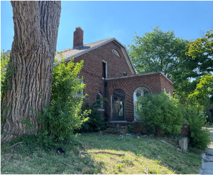
Site Photo 3, by Staff July 21, 2022: (South) Rear elevation, showing rear of sun porch and west elevation of the house.
