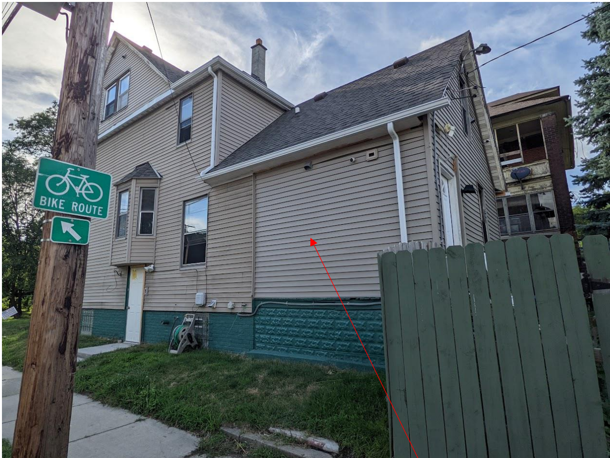
1402 Vinewood, current conditions, 7/27/2022 staff photos. Location of current project. Note work has been completed (slider windows have been removed and the area has been covered with vinyl to match adjacent)
