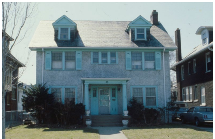
Designation Image, 1980: (Northwest) front elevation, showing slate roof, original porch and shutters.
