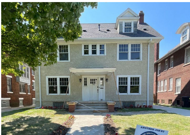
Site Photo 1, by Staff July 21, 2022: (Northwest) front elevation, showing installed asphalt roof.
