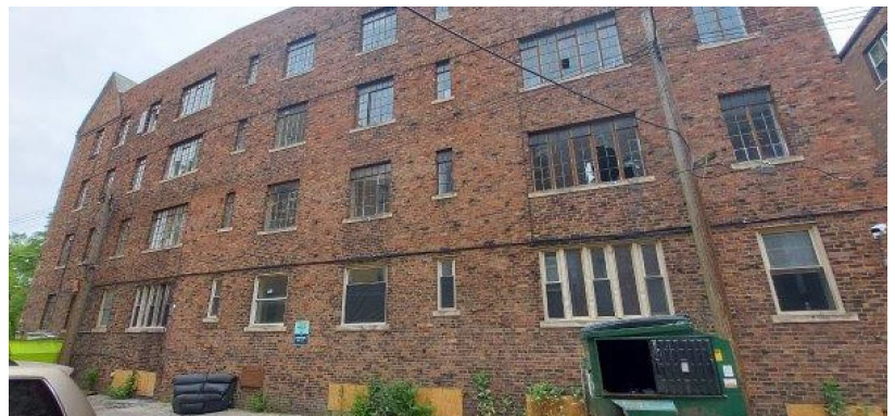
Site photo 4, by Applicant, on alley (west elevation), showing replaced windows on first floor prior to historic designation.
