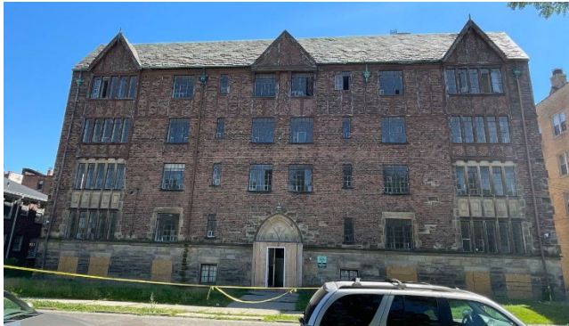
Site Photo 1, by Staff June 24, 2022: (North) Front elevation, showing original casement windows.
