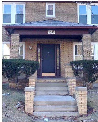
Front porch steps/piers, current appearance
