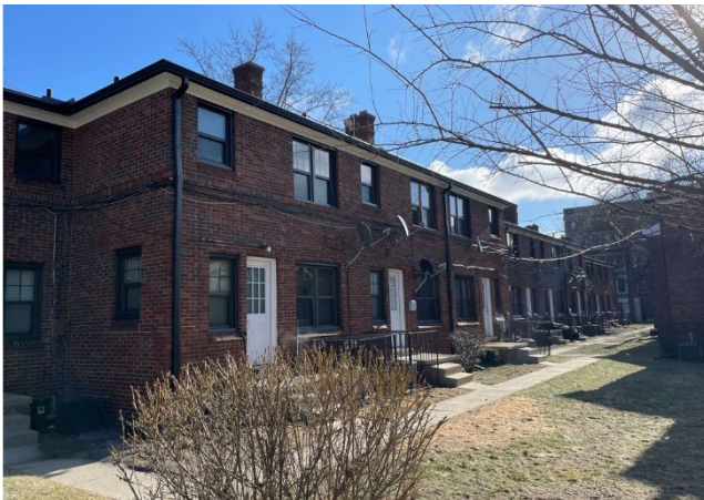
Site Photo 1, by Staff February 24, 2022: (Southwest) courtyard, showing vinyl window installation.
