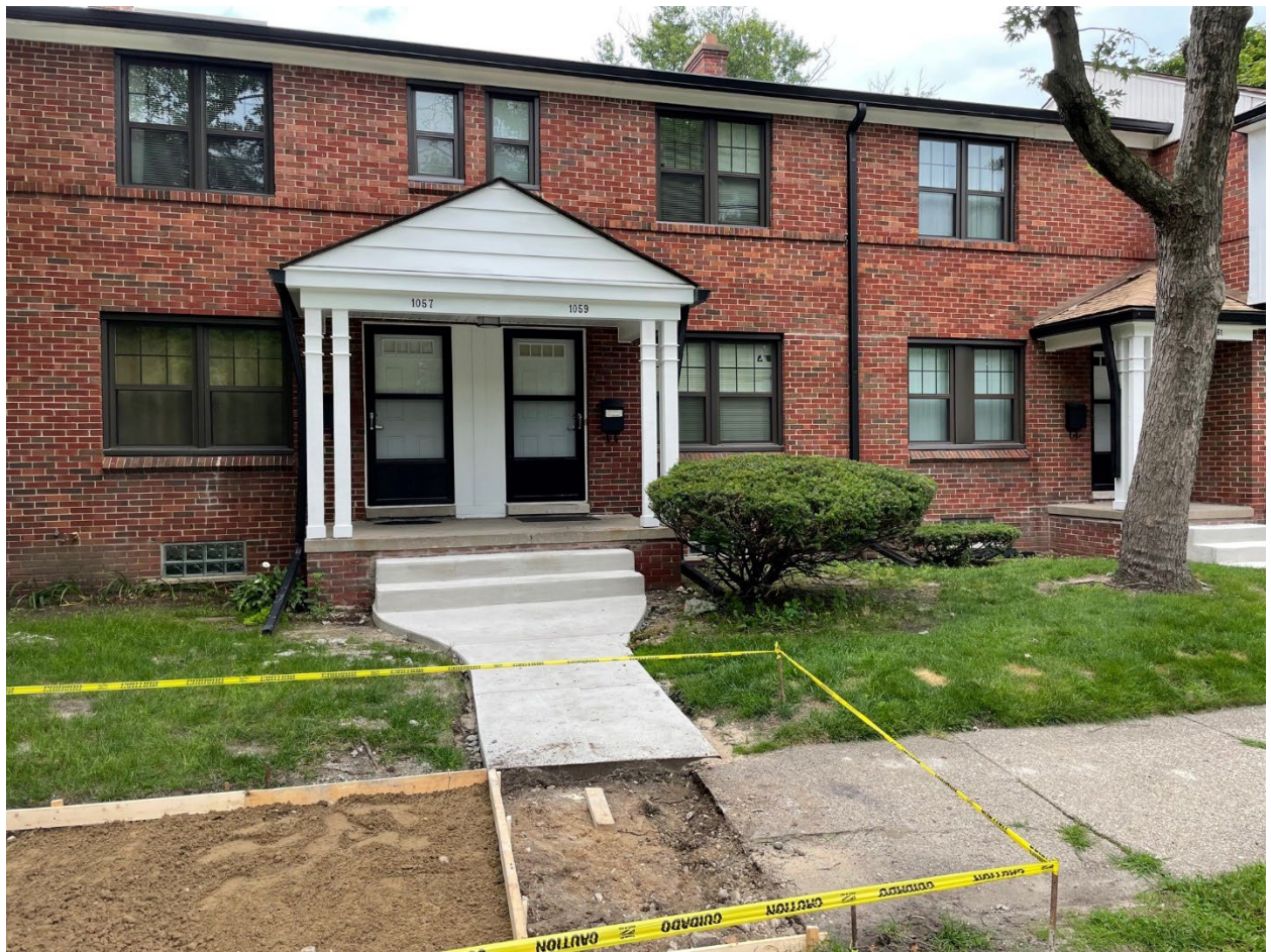
Photo 4: Phot showing new windows
