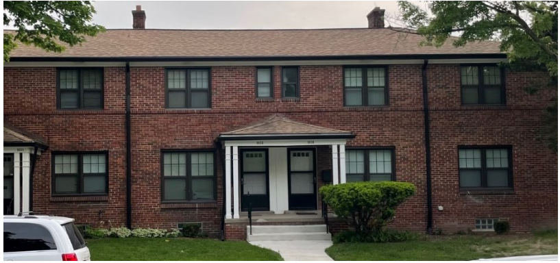
Site photo 6, by Staff, May 31, 2022: Covington (Northeast elevation), showing 6/1 between the glass vinyl windows, and 1/1 vinyl windows over the doors.
