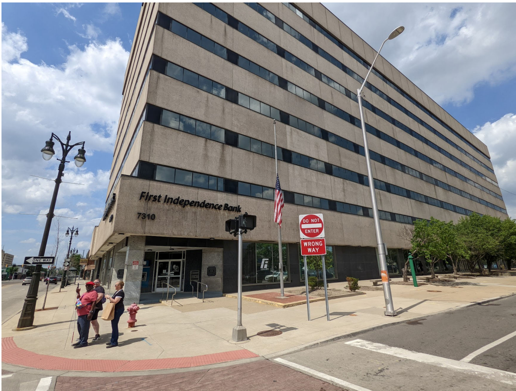
View of 7300 Woodward at East Grand Boulevard, looking north. Staff photo, June 1, 2022.
