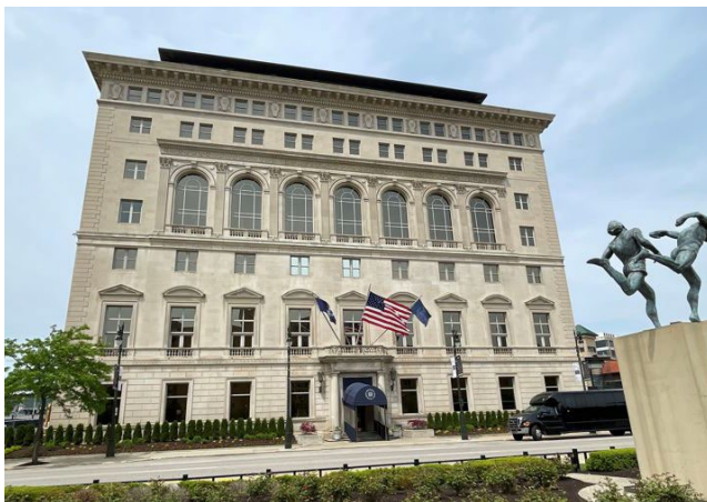
Site Photo 1, by Staff May 20, 2022: (South) front elevation.
