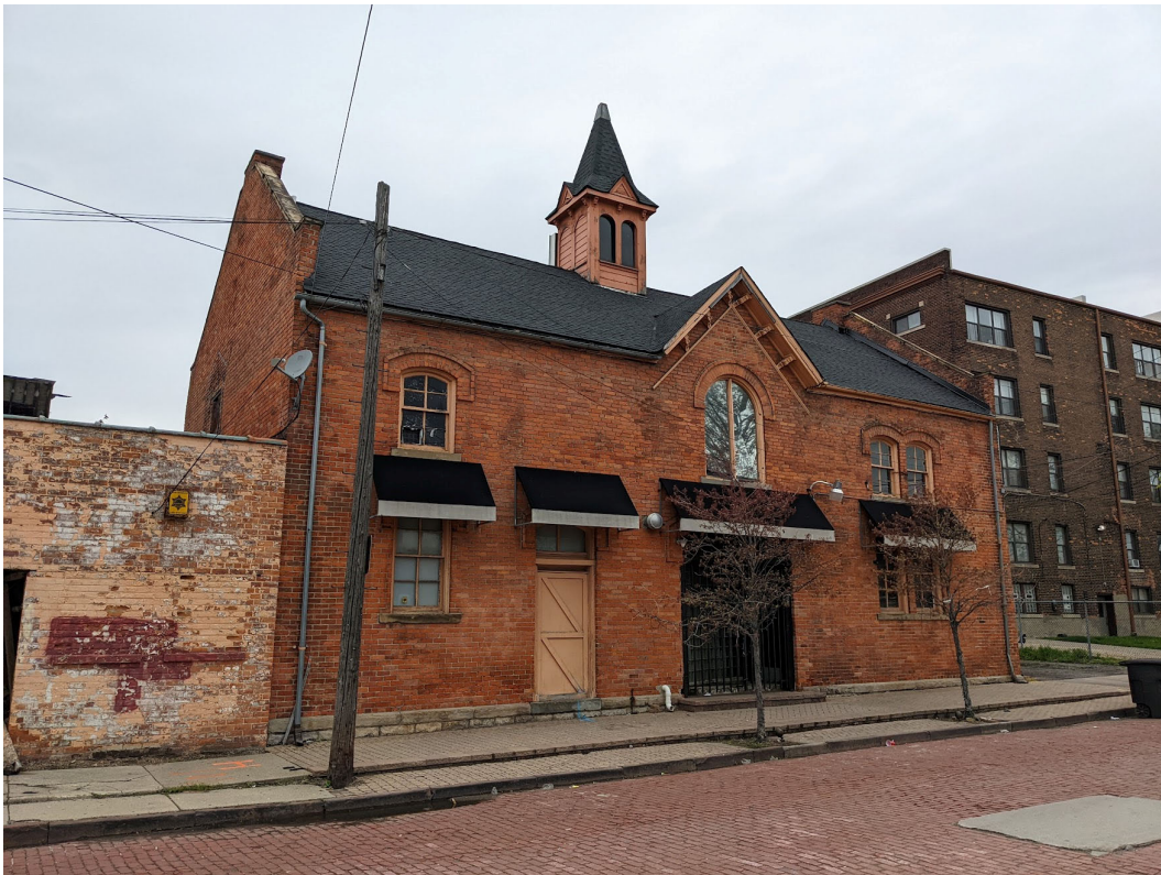
View of the single building in the McGregor Carriage House Historic District, erected circa 1885. Staff photo, May 6, 2022.
