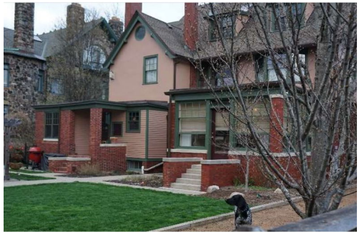
Site Photo 2, by Applicant April 2022: (Southwest) rear elevation showing proposed porch enclosure location (left).
