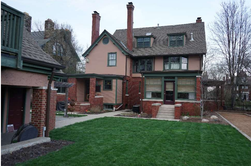
Photo 11 View of the full back of the house from yard looking east. Carriage house is visible at left. Porch to be enclosed is near center of the photo
