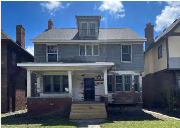
Site Photo 1, by Staff April 21, 2022: (Northwest) front elevation.
