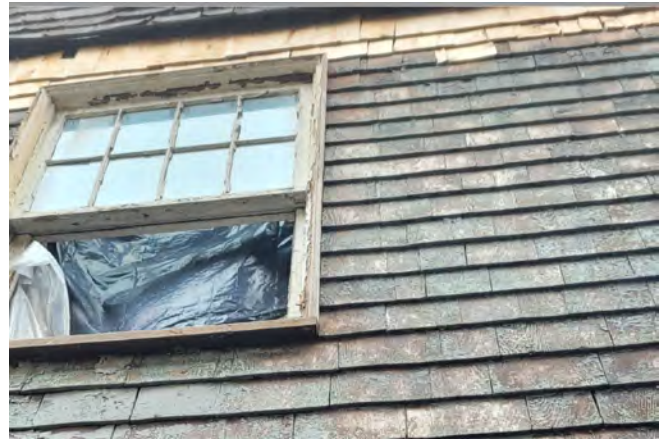
Site photo 4, by Applicant, showing completed siding work.
