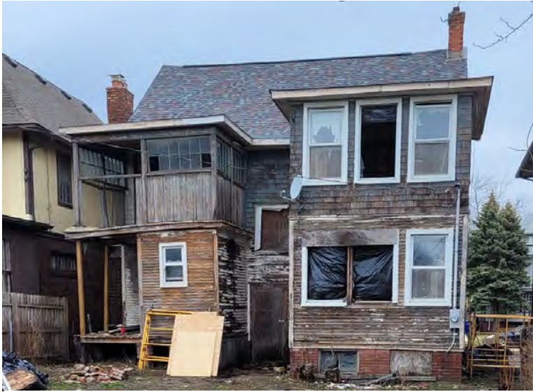
Site photo 2, by Applicant: Rear elevation (Southeast) showing current conditions and vinyl windows installed by a previous owner.
