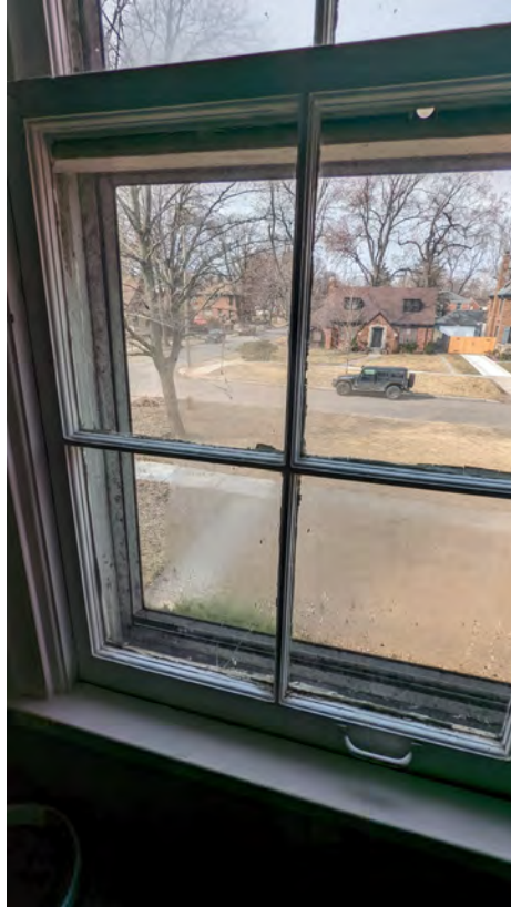
7. Upstairs bedroom 3 Exterior
