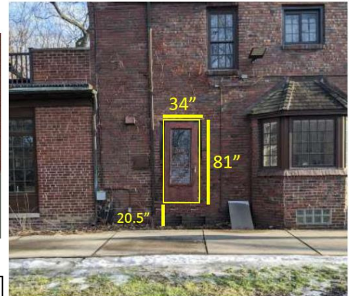
The door above is an actual snapshot of the door propped against the house. The colors are exactly as the finished product will be. The door has been digitally moved slightly up to show the finished install location.
