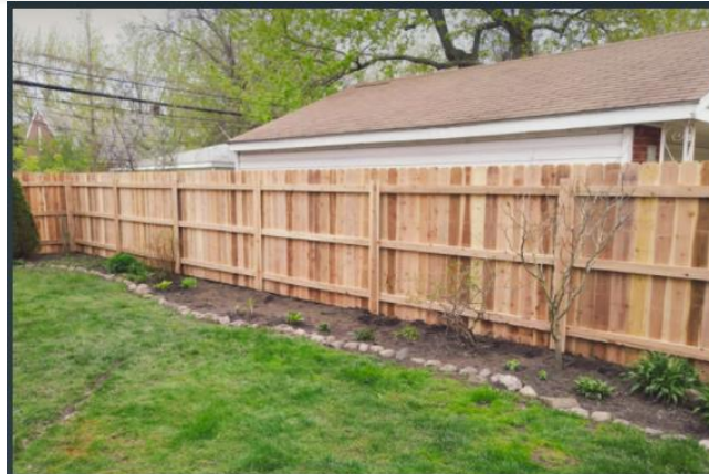
Cedar Solid-Board Fence (Interior View)
