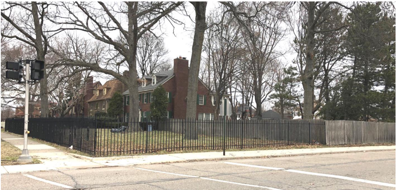
#2 NE corner of Burns and Charlevoix, March 23, 2022. Two material fence, multiple yard enclosures. Transparent fence at front yard, privacy fence beyond setback/rear yard. Both fences are only slightly set back from sidewalk. Important to note, there is no tree lawn buffer between Charlevoix and the sidewalk.
