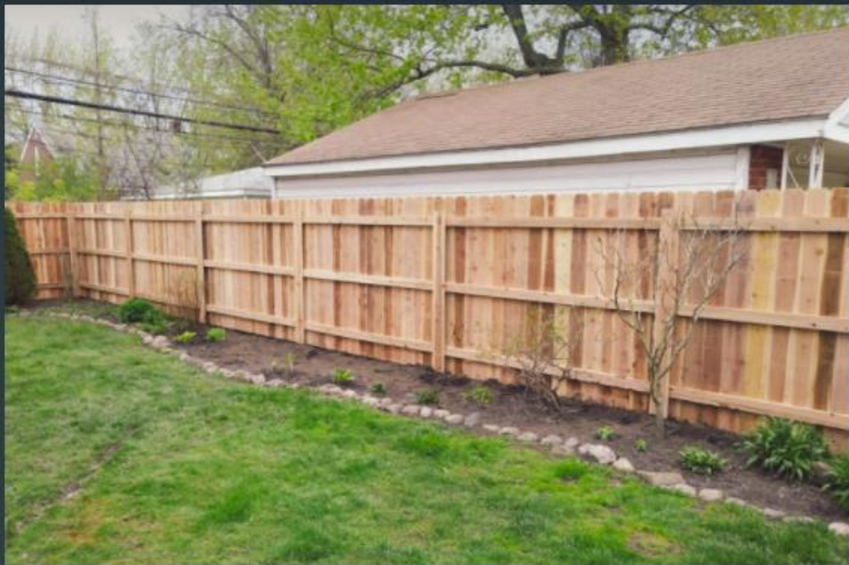
Cedar Solid-Board Fence (Interior View)
