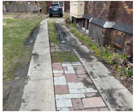
Site photo 8 by applicant, side elevation detail showing current driveway conditions..
