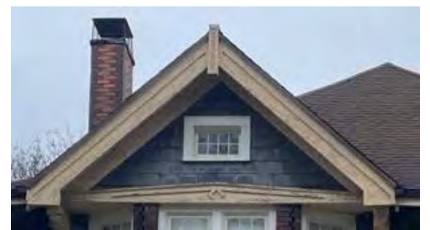
Site photo 7, by staff, March 25, 2022, front elevation detail of the dormer, showing slate siding.
