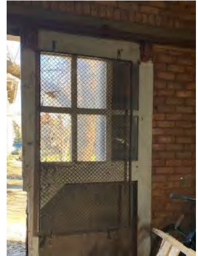
Site Photo 6, by Applicant, showing interior condition of the garage door.
