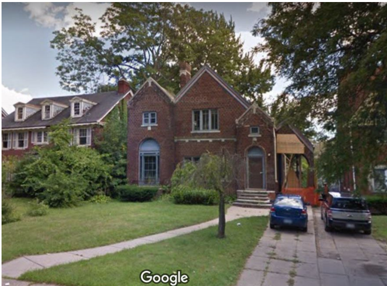
Site photo 2, by Google Street, August 2015: (Northwest) front showing original porte cochère shored up for future repair.
