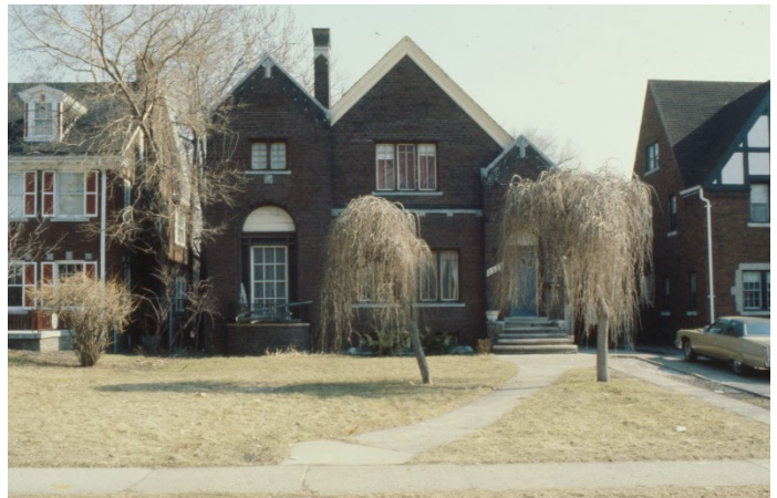
Designation Image, 1980: (Northwest) front elevation, showing original front porch and porte cochere (behind tree).
