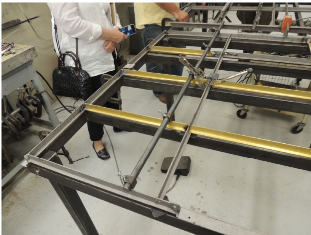
During restoration (installation of new members/Dutchman repairs)
