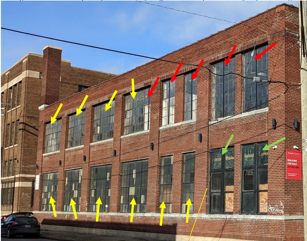
Above and below images: Non-historic steel sash windows indicated with red, historic steel sash windows in yellow, wood windows in green. Front and side primary elevations only. Staff recommends preservation of all yellow and green locations.
