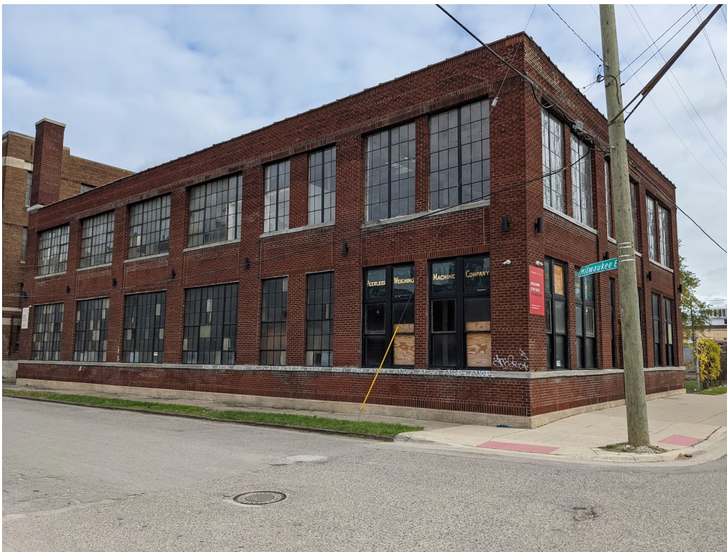
View of existing conditions at 603 E Milwaukee, corner of St. Antoine and E. Milwaukee. Staff photo, November 2, 2021.
