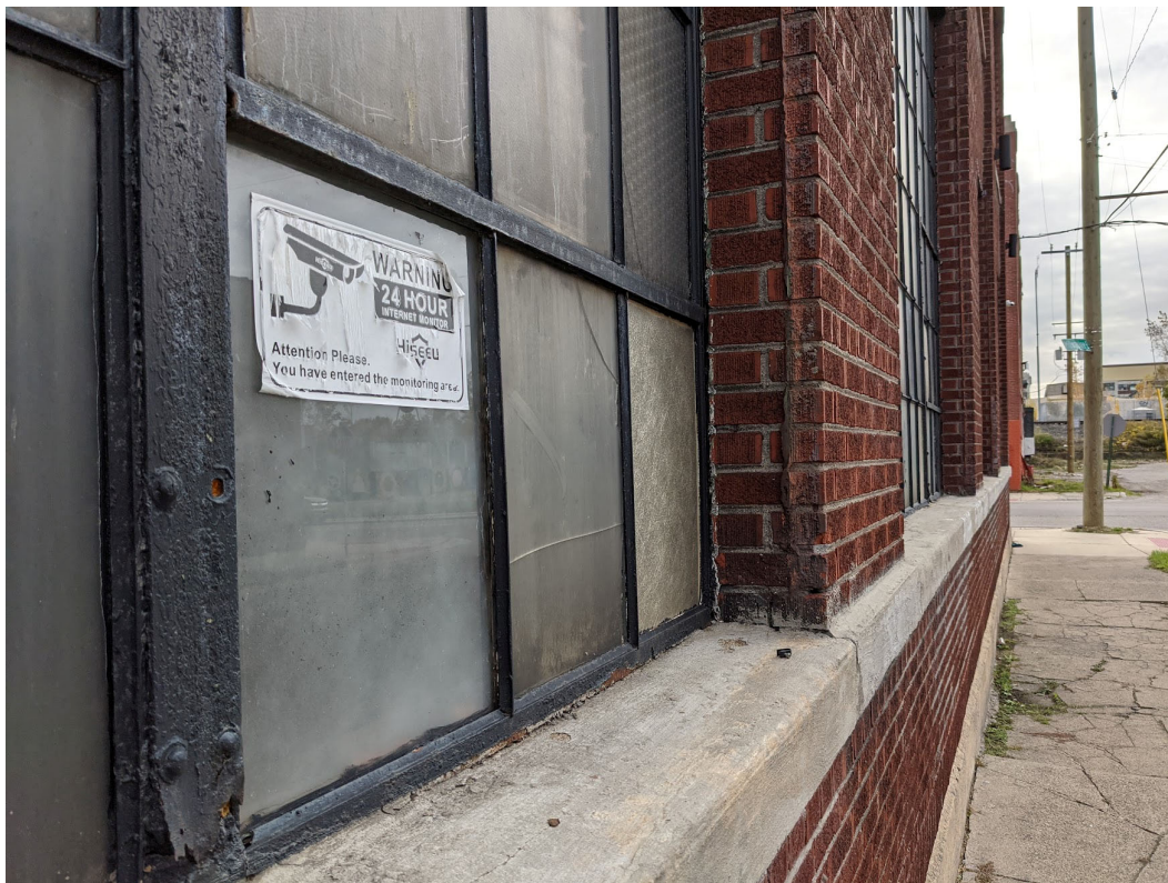
Detail view of steel sash windows and concrete sill/brick at first floor. Staff photo, November 2, 2021
