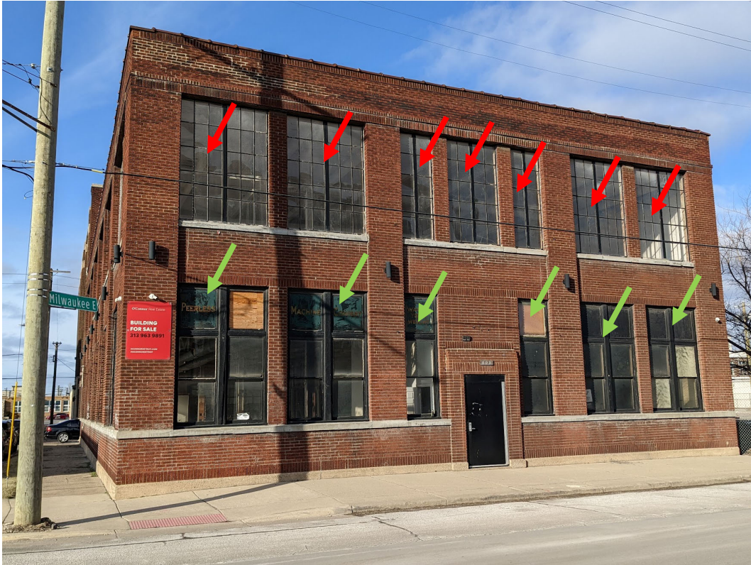
Above and below images: Non-historic steel sash windows indicated with red, historic steel sash windows in yellow, wood windows in green. Front and side primary elevations only. Staff recommends preservation of all yellow and green locations.
