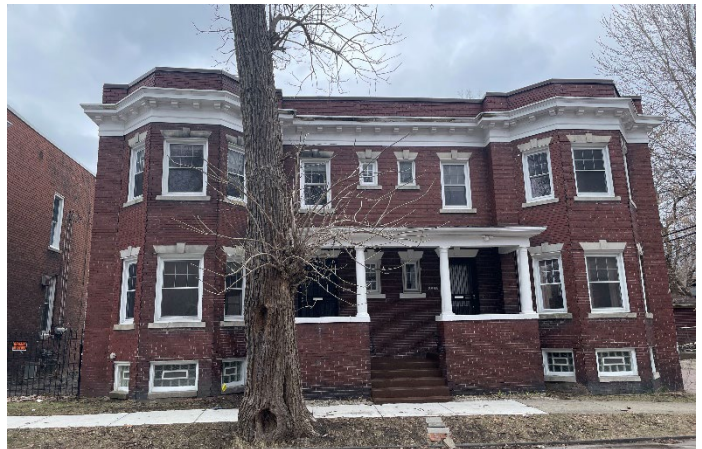
Site Photo 2, by Staff March 24, 2022: (Northwest) front elevation of 3821-3823 Shady Ln.
