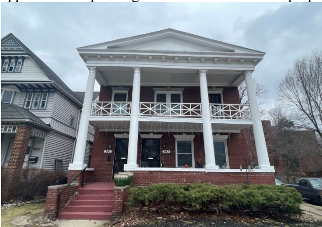
Site Photo 1, by Staff March 24, 2022: (Northeast) front elevation of 391-393 W. Grand Blvd.
