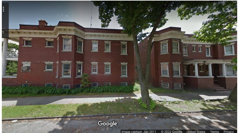
Site photo 5, by Google Street June 2011 (Northwest), showing original windows at both buildings.
