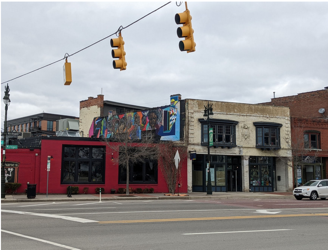
View of existing conditions at 1444 Michigan, view towards the north, Staff photo, April 1, 2022.
