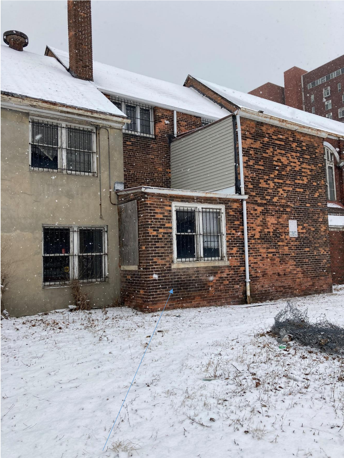
This wing will be demolished, with new wing to be built within the same footprint. The second-story portion of the new wing will be higher than the current. The existing brick will be reused to clad the new wing.
