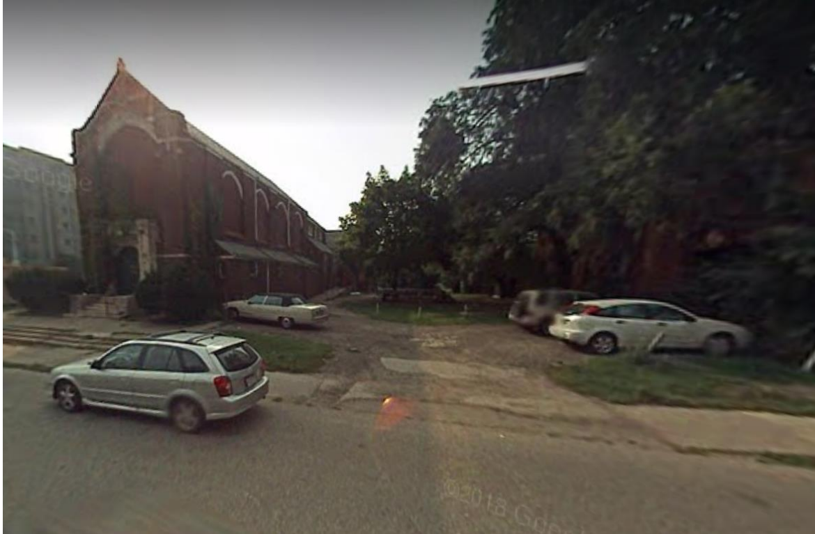
86 E. Forest, Google Streetview, 2007. Note presence of curb cut
