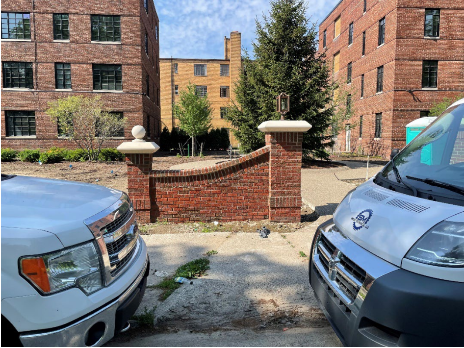
Photo 7: View of Central Courtyard from Street
