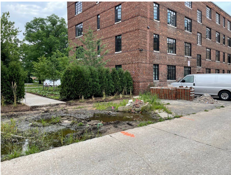
Photo 2: View of Right Center Area from Alley
