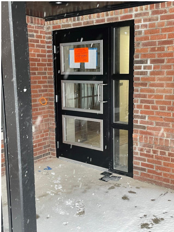
Photo 3: View of 885 Covington Entry Door
