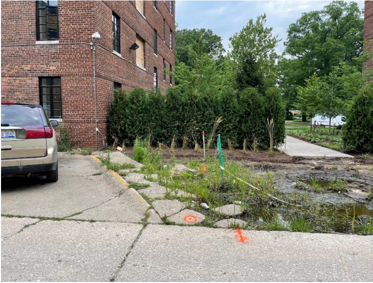
Photo 1: View of Left Center Area from Alley
