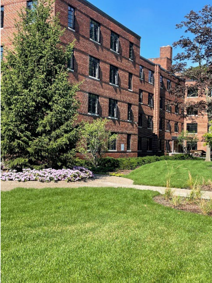
Photo 2: 931 Covington form Street
