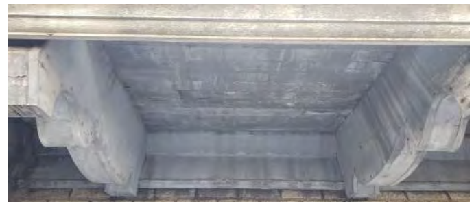
FIGURE A4.3 DECORATIVE WOOD EAVE IN FAIR CONDITION; (NORTH ELEVATION)
