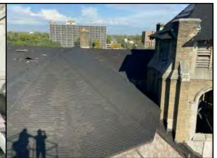
UPPER SLOPING ROOF AND OVERHANG IN MODERATE CONDITION
