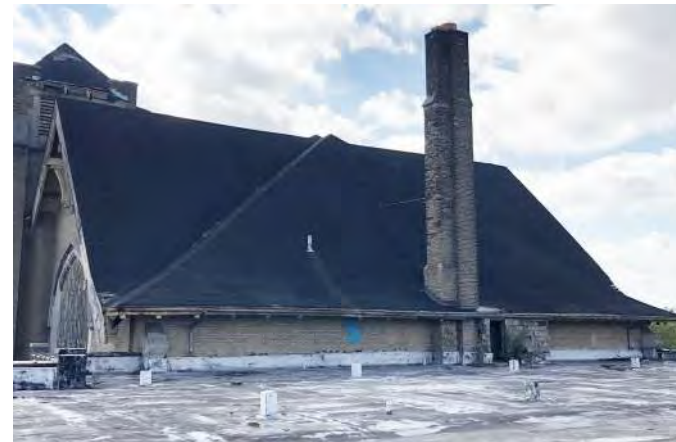
FIGURE A4.00 OVERVIEW OF NORTHERN SIDE OF THE CROSS GABLE ROOF
