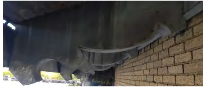
FIGURE 4.2 DECORATIVE WOOD EAVE, SIDE ELEVATION APPROX. LENGTH 3'-4"; IN FAIR CONDITION
