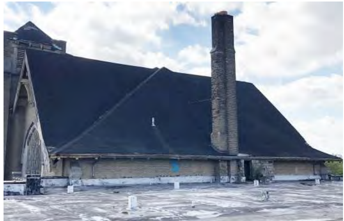
FIGURE A4.00 OVERVIEW OF NORTHERN SIDE OF THE CROSS GABLE ROOF
