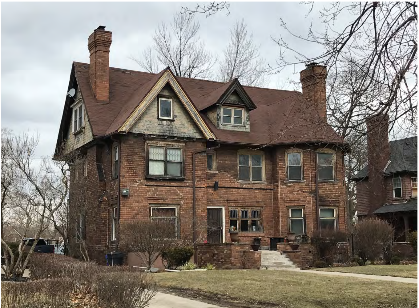
View of existing conditions at 235 E. Boston Boulevard looking northeast from E. Boston Blvd. Staff photo, March 8, 2022.
