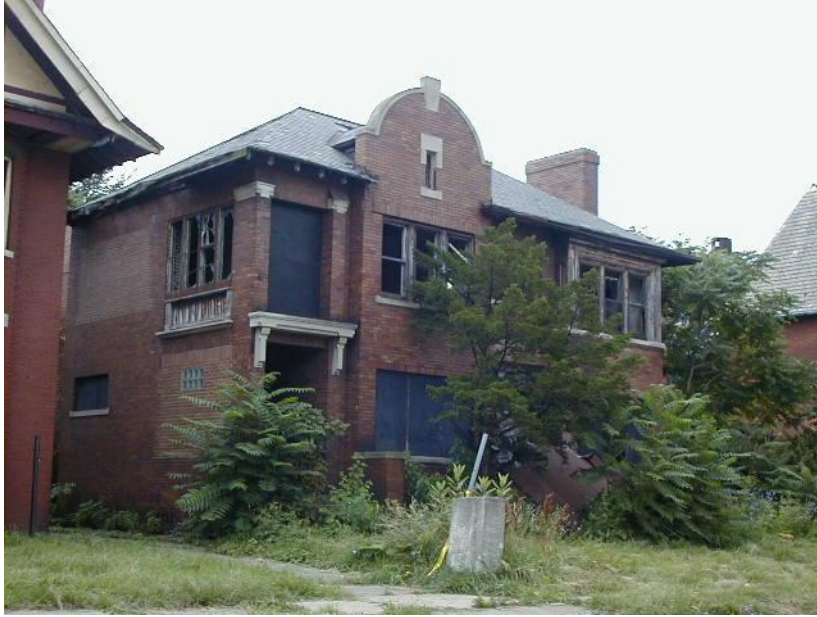
296 Eliot, photo taken in 2000, prior to rehab
