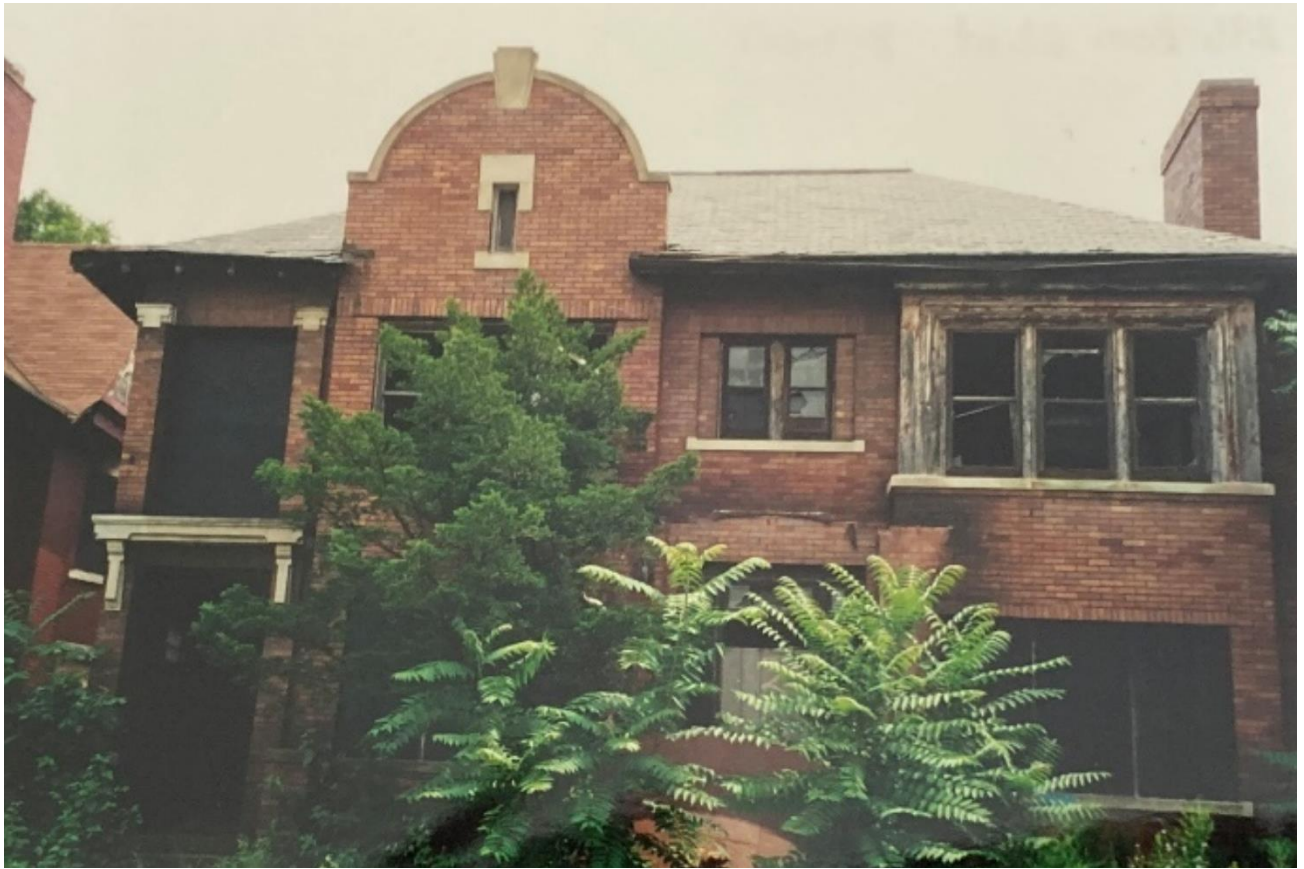
296 Eliot, photo taken in 2000, prior to rehab
