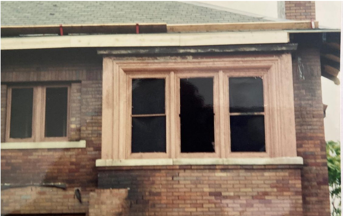
296 Eliot, photo taken in 2001, during rehab
