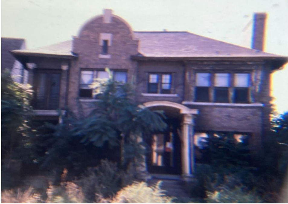
Designation slide. Appearance in 1980. Note window operation, light configuration and remaining surround at front-elevation, second-story western triple-sash window bay
