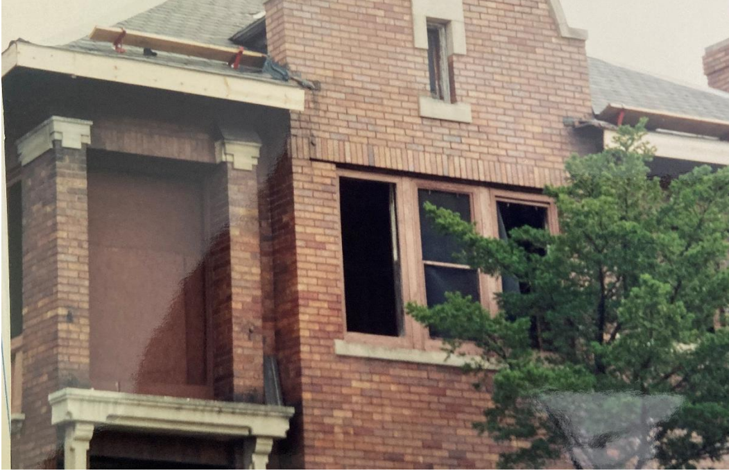
296 Eliot, photo taken in 2001, during rehab
