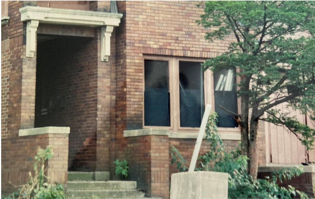
296 Eliot, photo taken in 2001, during rehab
