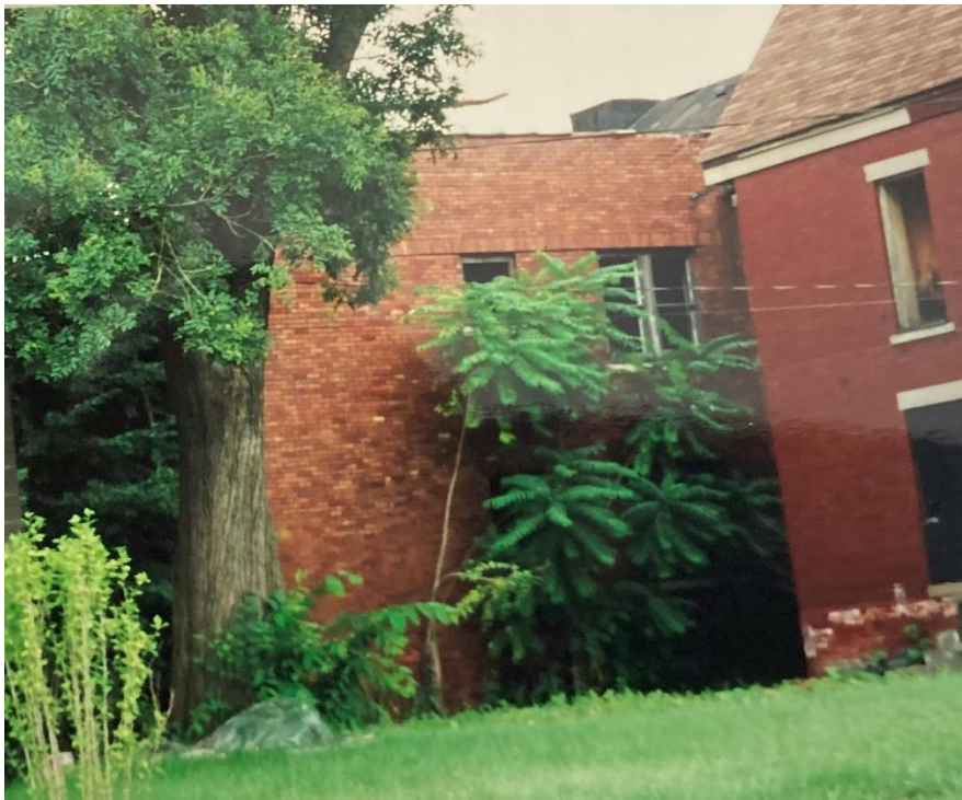
296 Eliot, photo taken in 2000, prior to rehab
