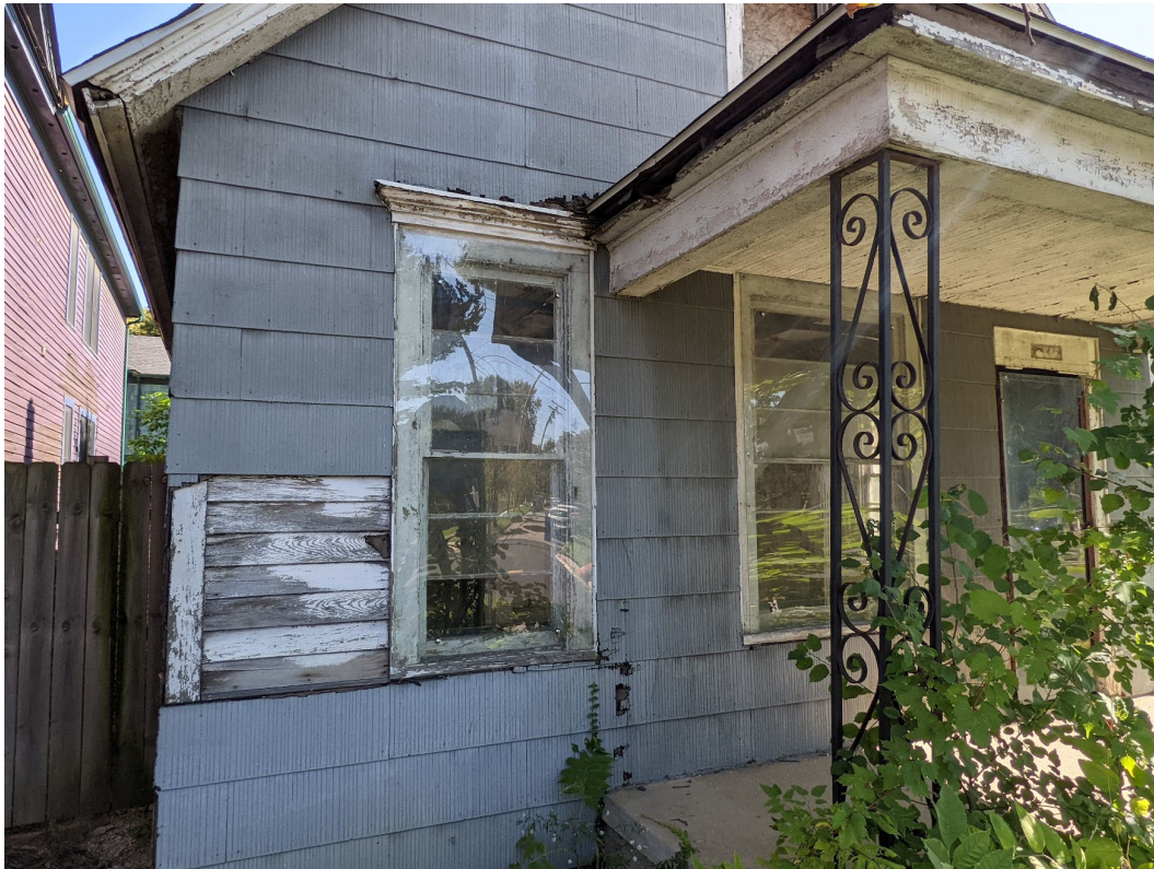
Front view of 1532 Van Dyke, looking east. Staff photo, October 1, 2021.
