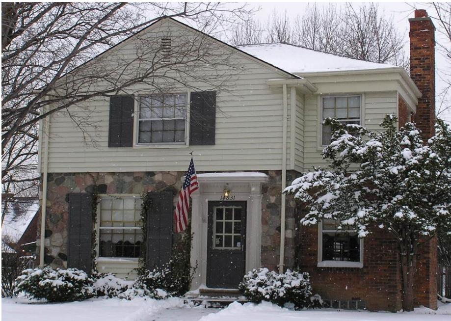
14831 Warwick designation photo, 2007. Photo shows original windows, all of double-hung operation.
